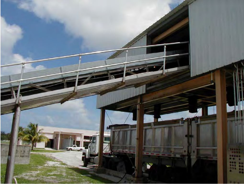
ECRWWTP Truck Loading
