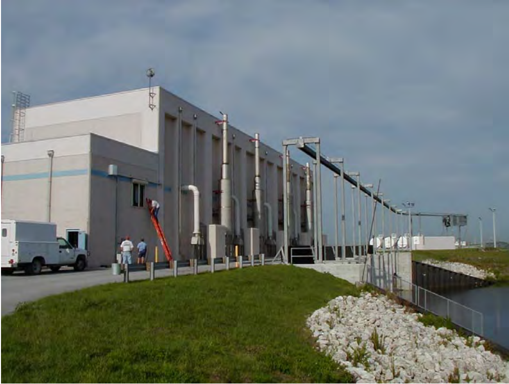
SFWMD Pump Station 319
