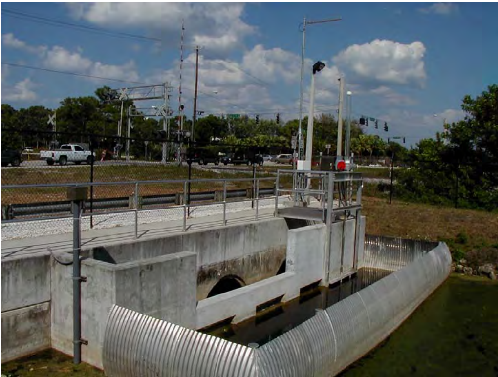
NPBCID Water Control Structure
